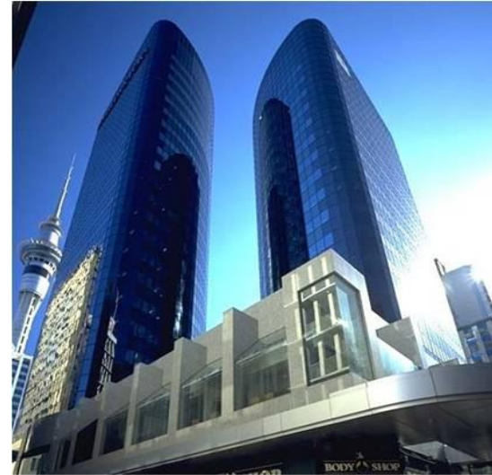
National Bank Centre Auckland
