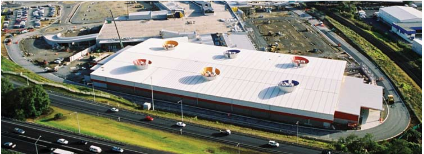
Left: Tiling of internal mall walkway. Right: Pedestrian walkway on eastern side. Bottom: The Warehouse.
